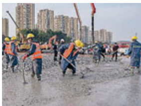
Lavori in tempi record.
